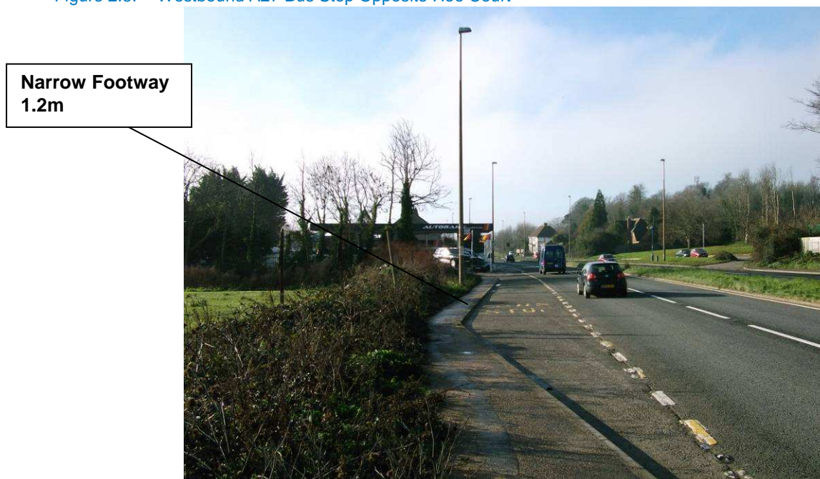
Figure 2.5: Westbound A27 Bus Stop Opposite Hoe Court
